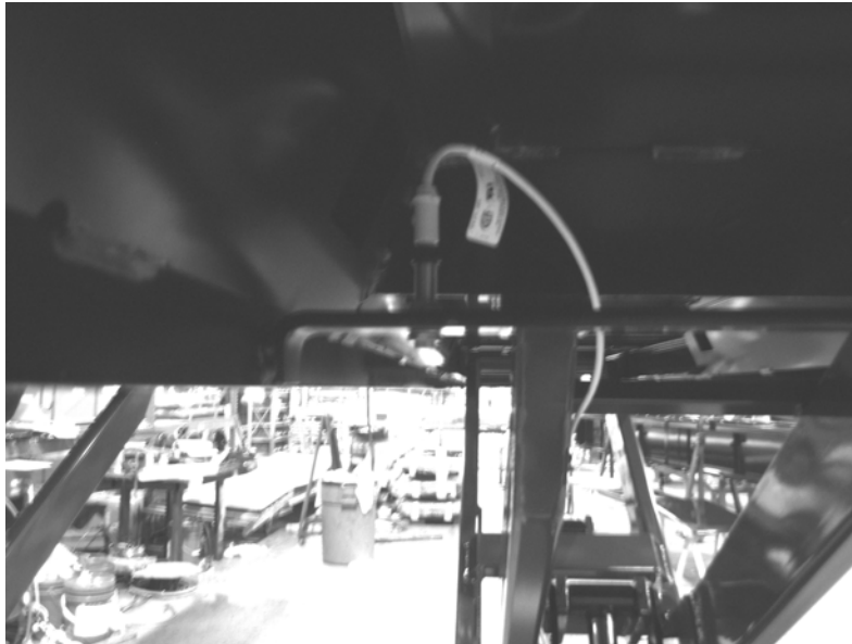
Figure 9b – Equalizing proximity sensor Under front of deck.
